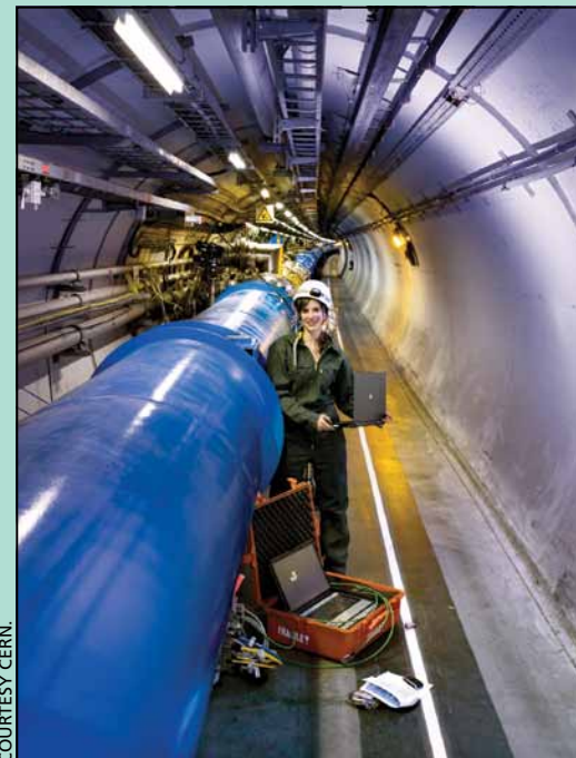
C. An engineer checks the electronics of the instrumentation under a dipole magnet in the Large Hadron Collider.
